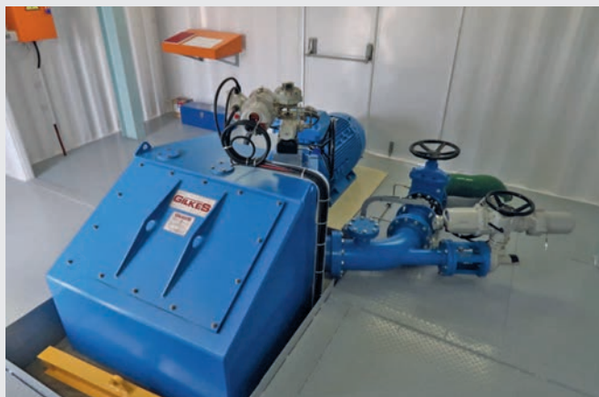
The Gilkes 12” Turgo Impulse turbine supplied for AngloGold Ashanti’s Sadiola gold should generate around 150 kW at 400 V
