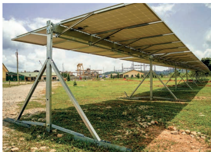
Cambridge Energy Partners' Nomad is a prefabricated and re-deployable solar generator with single-axis tracking technology
