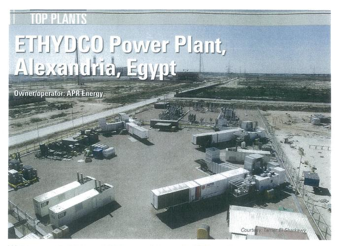
Within roughly 90 days, APR Energy set up a 60-MW turnkey power plant—complete with novel natural gas filtration and compression solutions—to support the operations of a massive Egyptian polyethylene plant until a bigger, permanent power plant can be built.
